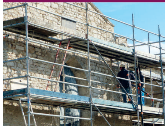
1. Restauration des jointements © M. Bompard
